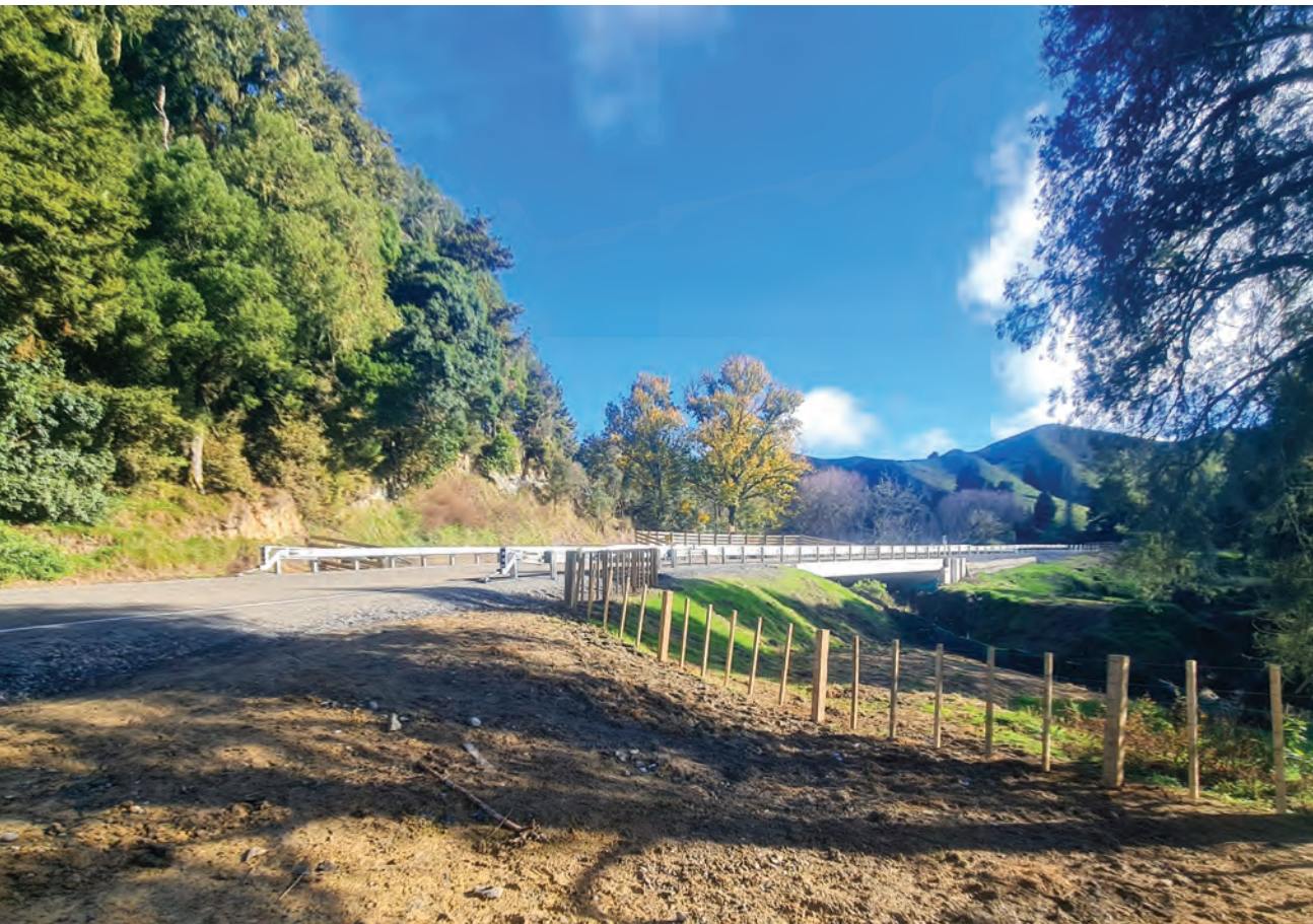
A new 20 metre bridge across the Kururau Stream is helping future-proof the Forgotten World Highway.
