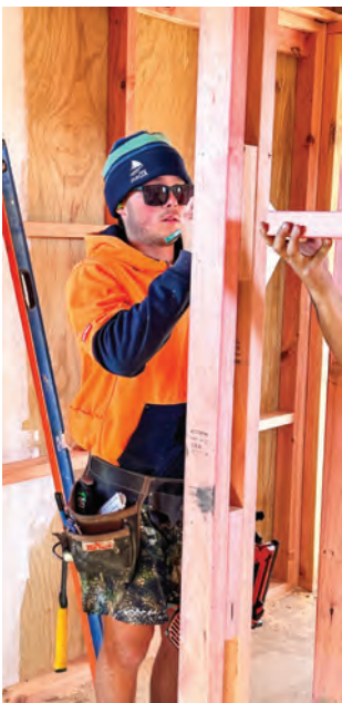
Bailey Feek working on internal framing in the bathroom.
