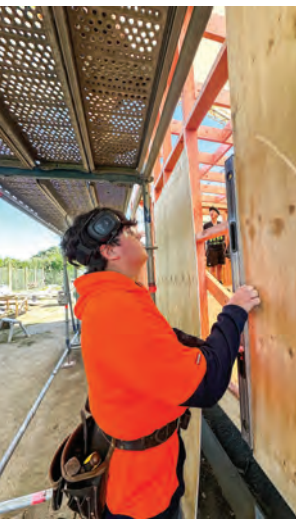
A side on view of Jaden Dougherty who is levelling up a sheet of bracing plywood.
