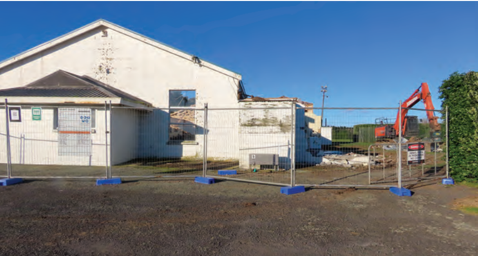
Work begins on demolishing the Manaia Sports Complex.
